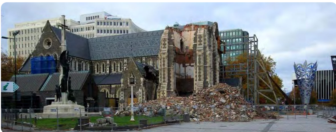
Fig. 1 Damage to Christchurch Cathedral in the heart of the city, including collapse of spire ( https://picasaweb.google.com/RossBeckerNZ/2011April27IntoTheChristchurchRedZone#slideshow )
