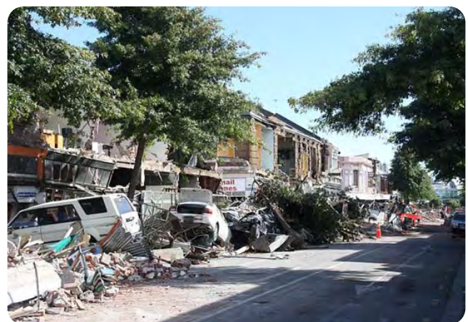
Fig. 4 Damage in a central Christchurch street (Photo: John Taylor)
